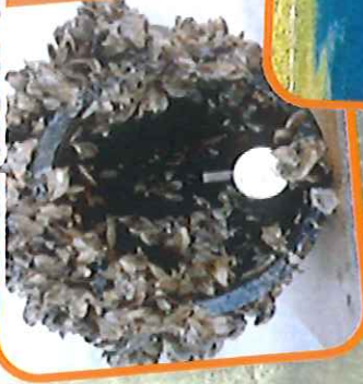
Quagga mussel growth on ABS pipe from Lake Mead, Arizona
